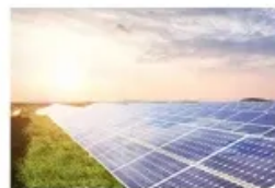
Energy Storage System
