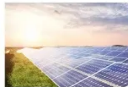
Energy Storage System
